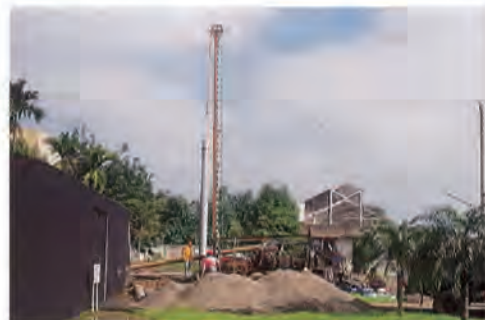
▲ 凿井工程 Well drilling engineering
