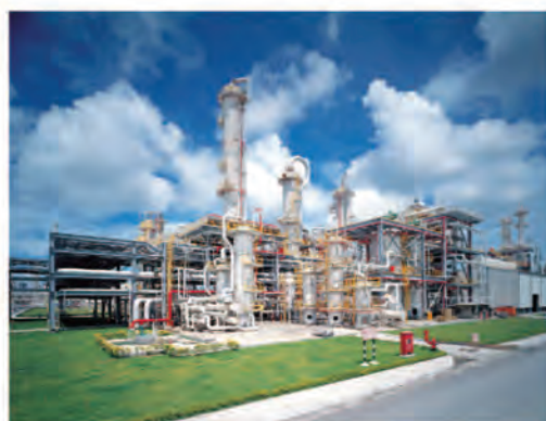
▲化学工厂 Chemical factory
